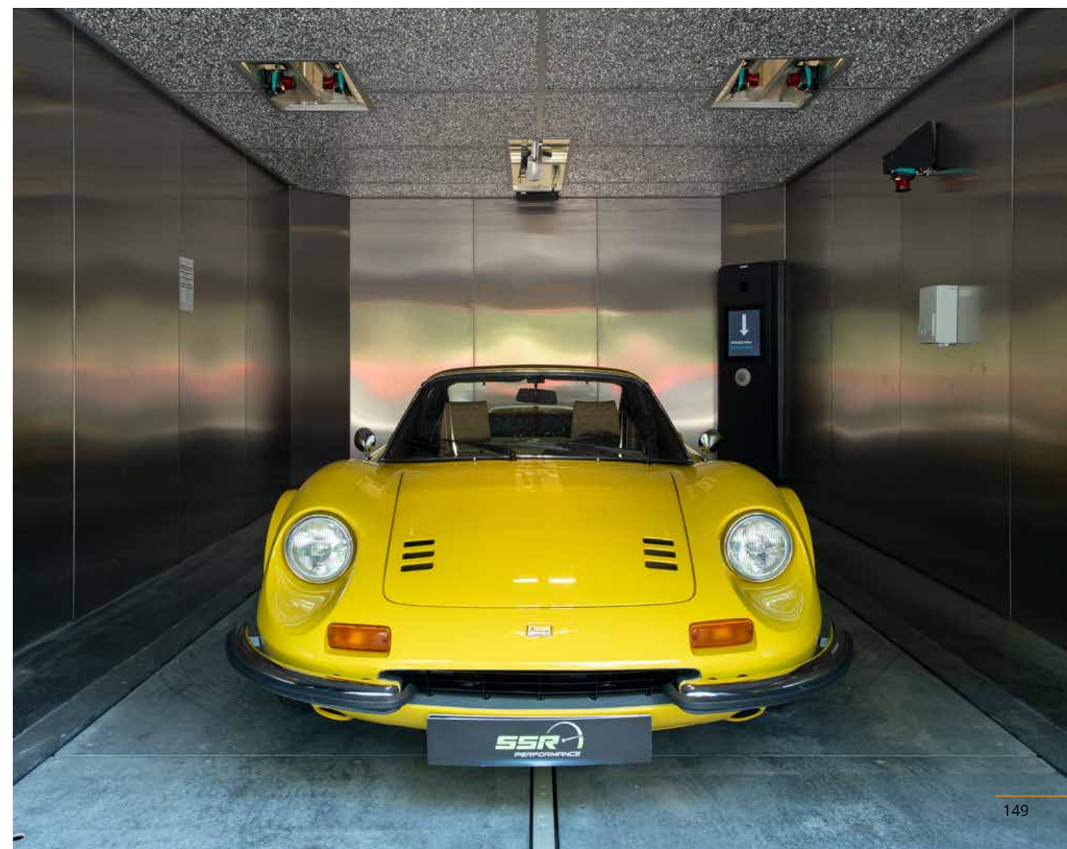
Lift ceiling made of Alusion™ by Cymat Technologies, AL-FG-12.7-LG-2S (large cells, open both sides), project: SSR Performance Munich, photos: Henning Koepke
