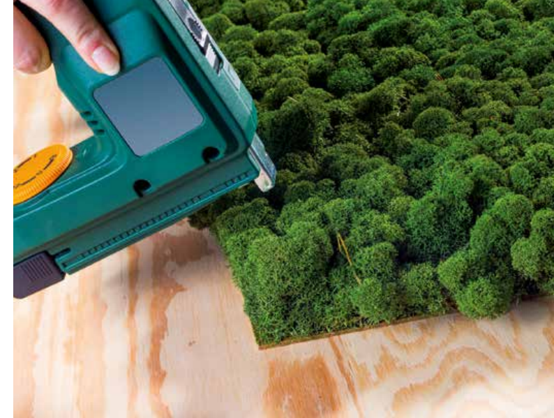
The moss boards can be stapled (for example, with an electric staple gun), screwed or glued directly onto a wooden substrate. Photo: KOMPE IMAGES
