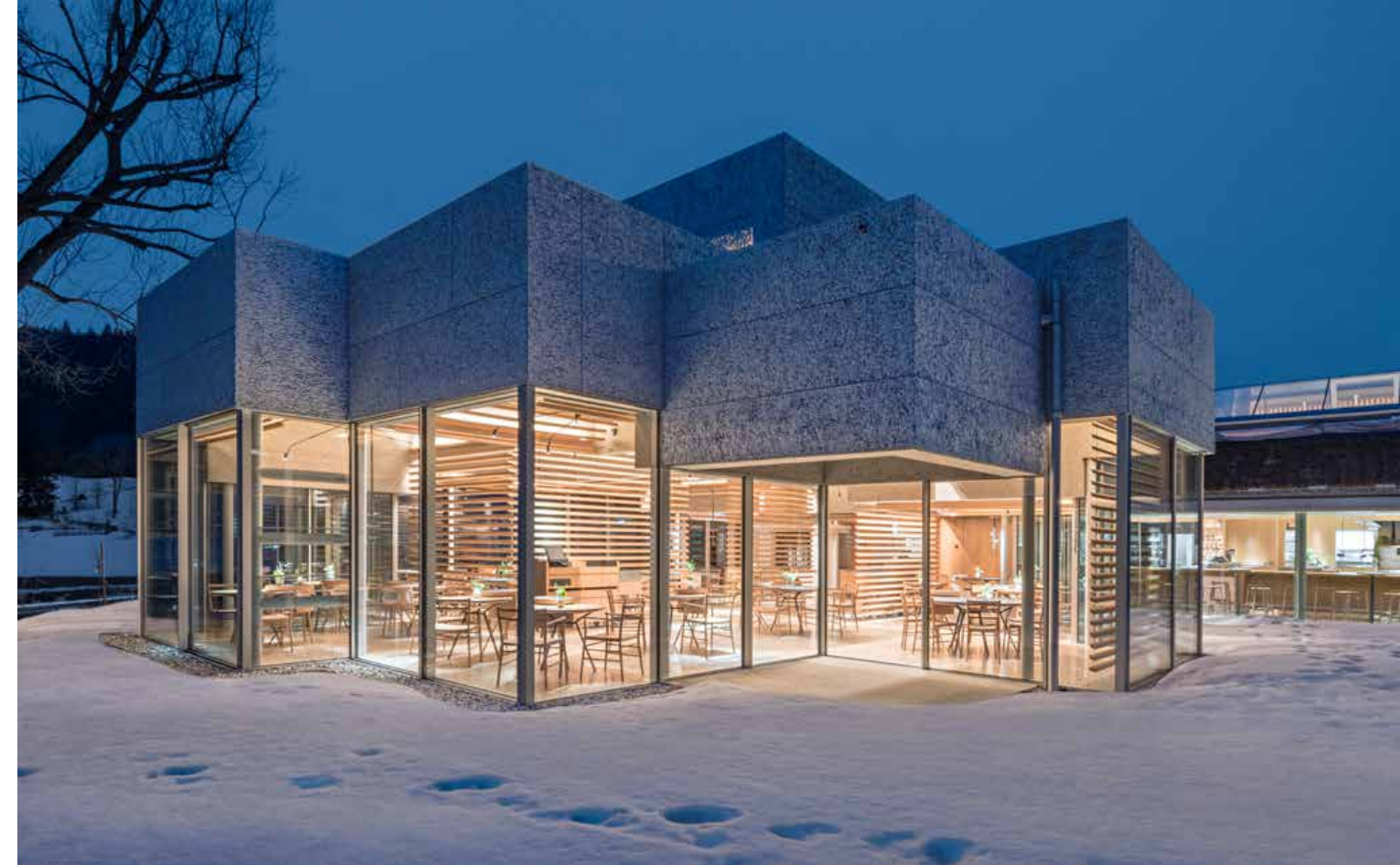
Traditional cabin aesthetic contrasted with modernity in aluminium and glass Alusion™ by Cymat Technologies, AL-FG-12.7-LG-2S (large cells, open both sides) Project: glazed pavilion at the Pogusch Country Inn in Turnau (Austria) with live kitchen, realisation: Alois Perwein GmbH, photos: Hertha Hurnaus
