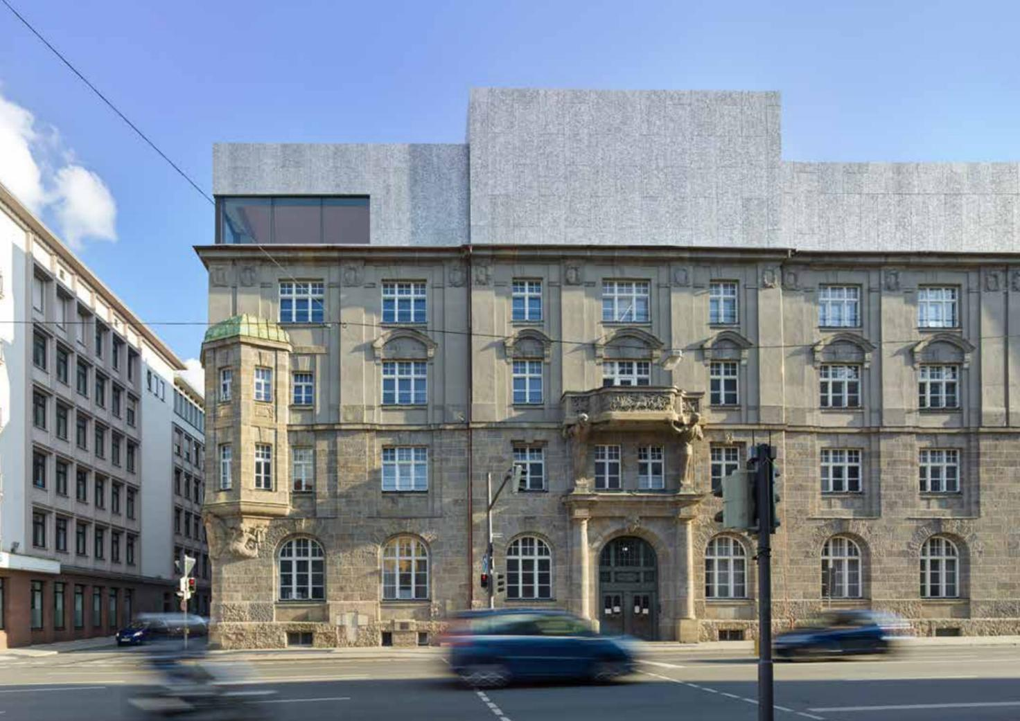
Alusion™ by Cymat Technologies, AL-FG-12.7-LG-2S (large cells, open both sides),
